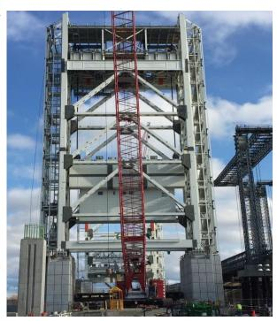
Weight of counterweight 700 Tons Lowering distance 135' Weight of sheave 80 Tons Lowering distance 250'
