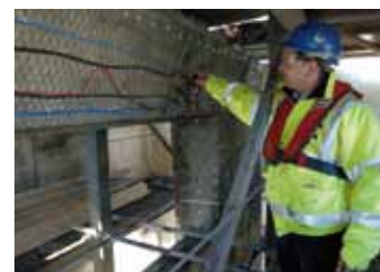
Cathodic corrosion protection (Foreva® CP Mesh Solution)
