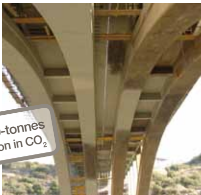
Maameltein bridge repairment - Lebanon
