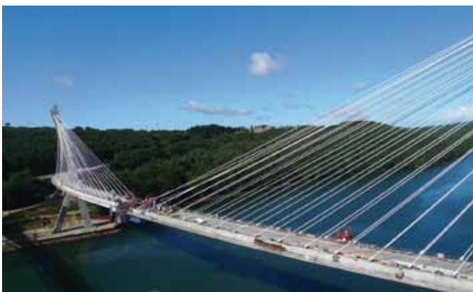
Stay cables, Terenez Bridge - France
