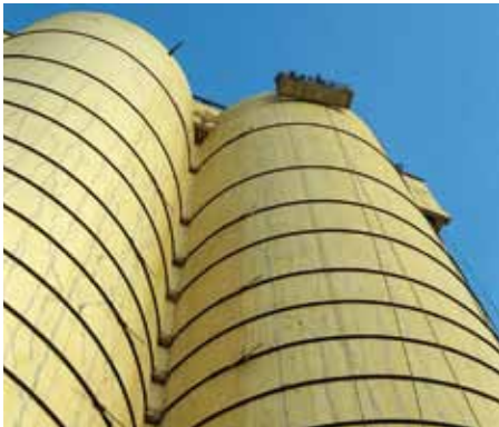
Industrial structures repair
