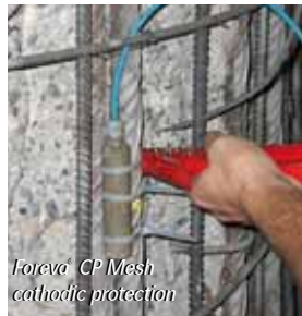
Electrochemical treatment against corrosion
