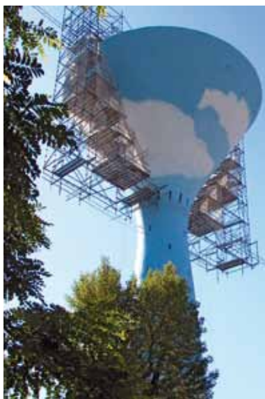
Water tower repairment with Foreva® solutions
