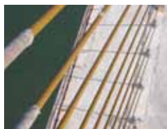
High fatigue resistance, compact sheath stay cables
