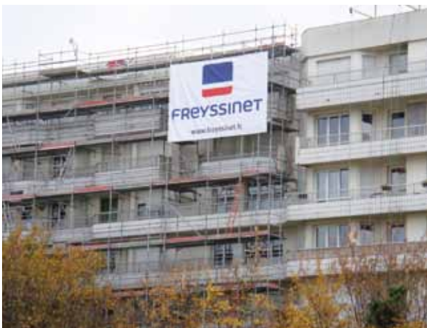
Balcony reinforcement - France
