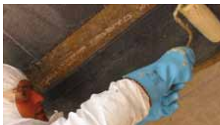
Carbon fiber fabric composite (Foreva® TFC Solution) for reinforcing structures
