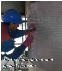
Foreva® CP Mesh cathodic protection
