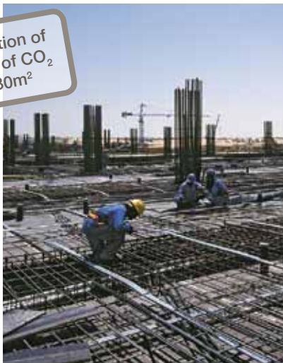
Prestressed floor - Dubai
